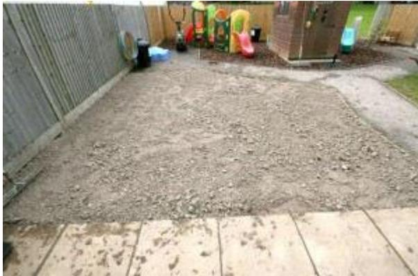
Make sure the Type 1 or Grano Dust is evenly spread and smooth off any lumps with a rake. The Type 1 should be raked level with top of the timber perimeter edging and then compacted with a wacker plate. Compact the Type 1 with a wacker plate and blind off with a thin layer of Sharp Sand. If using Grano Dust, no Sharp Sand is required, Grano Dust when compacted gives a smooth enough finish
