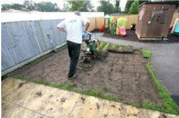
Remove the existing turf and soil using either a turf cutter or shovel. It is best to remove the turf to a depth of 2 – 3.5 inches. Free draining lawns will require a 2-inch base, whereas poor draining lawns will require a 3 to 4 inch base.
