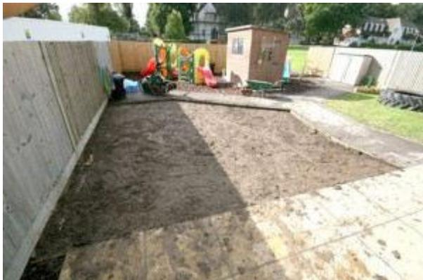
With all turf removed, the area is ready for the sub-base to be installed. The area should be edged by a timber frame, or concrete haunching, which provides a firm edge to hold the base material in place and a secure fixing point for the artificial grass. The timber edge should be fitted approximately 10mm below the surrounding level, depending of the pile height of your chosen artificial grass.
