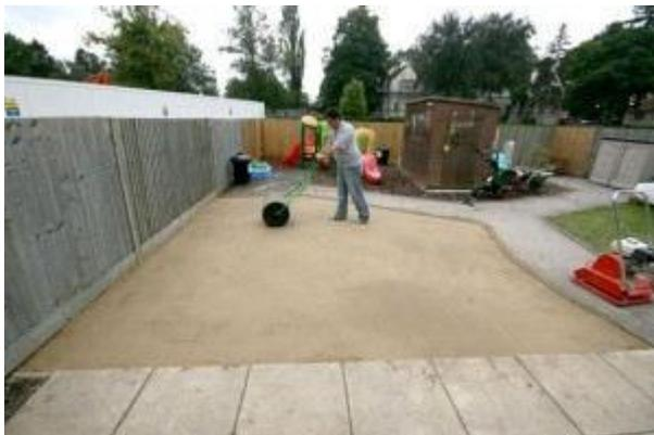
When using Grano Dust no sharp sand is required so top of compacted surface should be level with top of timber edging.
