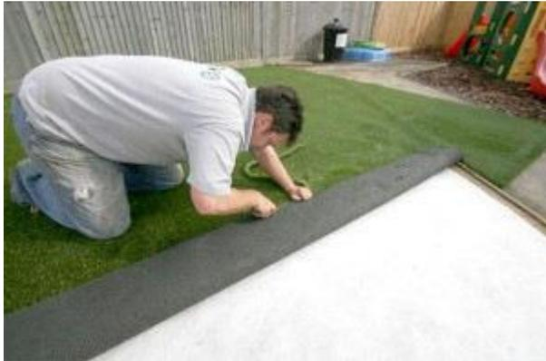
Lay the artificial grass out and leave to settle flat. Once you are happy that the grass is flat and settled, you can then cut it to shape using a sharp Stanley knife. Blades will need to be changed approximately every three metres of cutting.
