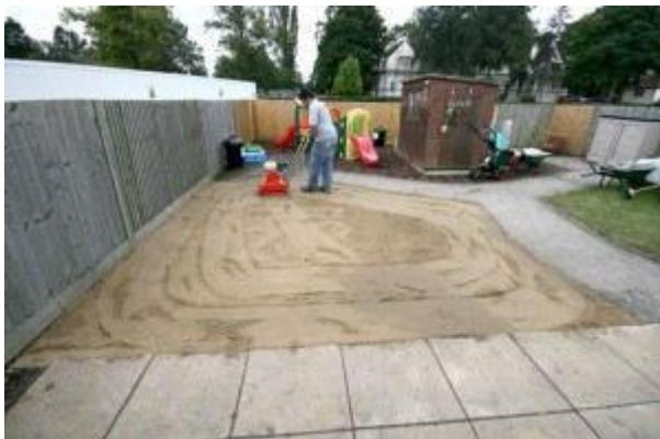
Using a wacker plate, make sure that all the Type 1 is compacted to a smooth finish. This should lower the Type 1 to approximately 10mm below the top edge of the perimeter timber. Now spread on the sharp sand and compact with a wacker plate, screed off to a smooth finish level with the top of the timber edging.
