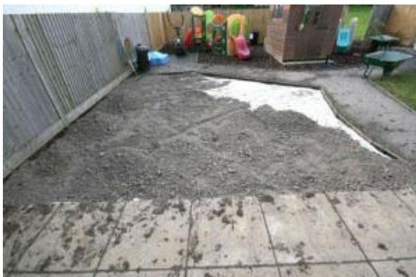
Install the first layer of geotextile weed membrane on top of the soil. This will prevent the sub-base sinking into the mud. It is best to fill the area with Type 1, sometimes known as MOT (crushed stone) or Grano Dust. For Clay or Boggy soil use between 65-100mm of Type 1, for free draining soil 50mm. A Grano Dust base of around 40mm will be sufficient.
