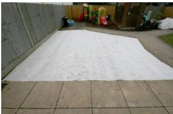
Install the second layer of geotextile weed membrane and secure to the top of the timber edging with screws or staples. This will prevent any weed growth. Use a Stanley knife to cut the membrane to the required layout.
