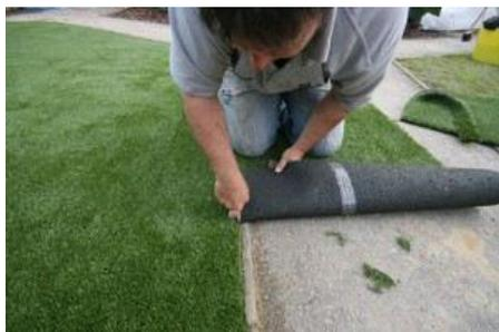
Now you can trim the edges. This is easiest done using a sharp Delphin knife. Change blades regularly for ease of cutting – this will result in a better quality installation with cleaner joins and edges.
