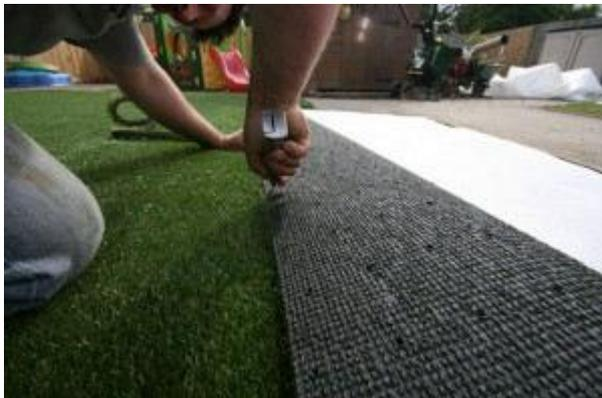
When joining two pieces of grass together, cut evenly down the side of a stitch line on each roll of grass, perhaps 1 or 2 stitch lines in from the edge of the roll. Butt the two pieces together and check the join. It is quite possible there is still some trimming to be done.
